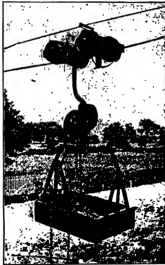
FIG. 134.—Installation on Telfer System: Portion of Line with Truck and Carrier.
